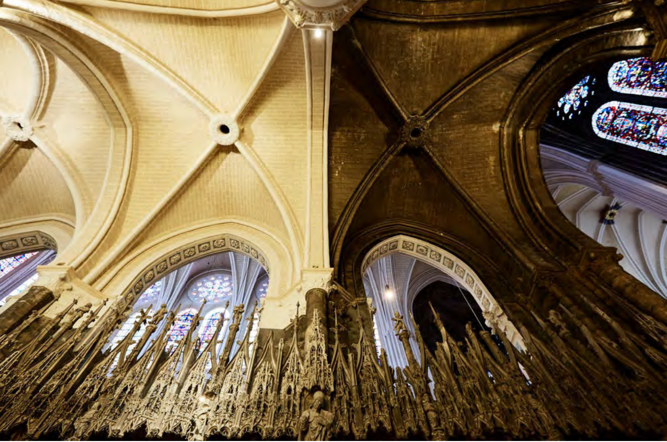
Figure 20: Frankenberg, R. The contrast between the restored and untouched sections of the cathedral is stark , 2017. Web. The New York Times , 25th February 2020.
