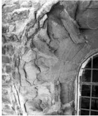
Figure 15: Uncredited, Spalling due to thermal shock in stonework from a monastery in Lobenfeld, Germany . Photograph. Undated. Image sourced from Hajpal, M. Fire Damaged Stone Structures in Historical Monuments. Laboratory Analyses of Changes in Natural Stones by Heat Effect . Web. 25th February 2020.
